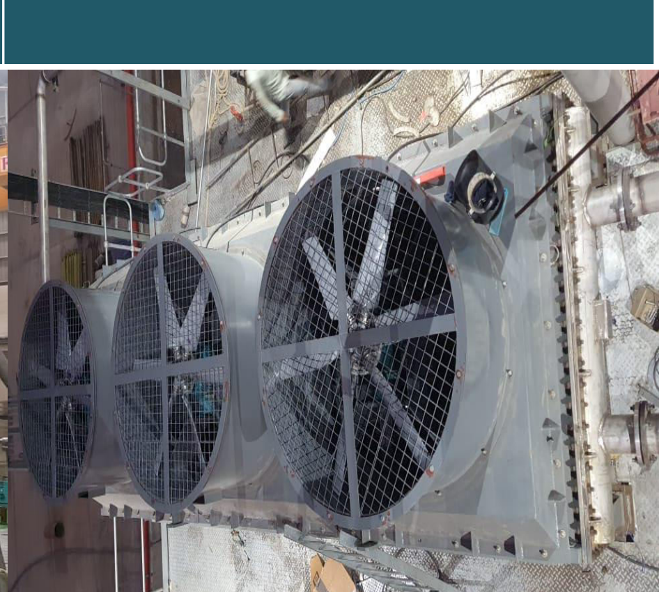
STAINLESS STEEL ACHE ETHANOL EXTRACTION, KPR SUGAR & APPARELS LTD,
